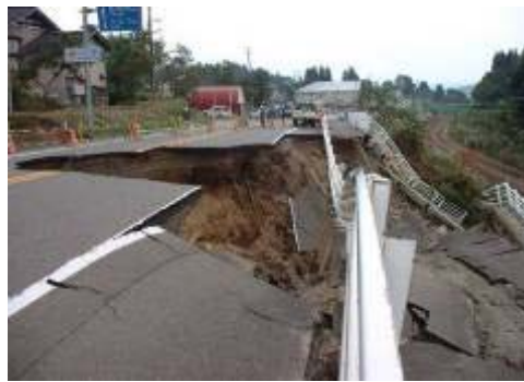
Photo 1 – Example of destruction of roads by the Niigata earthquake
