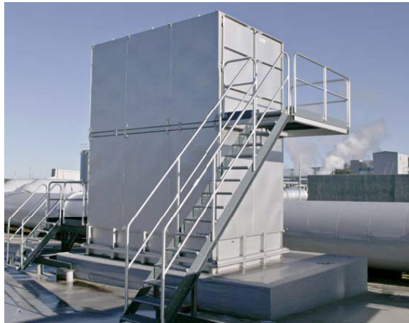
Figure 5 – New baffle-type BVN silencers
