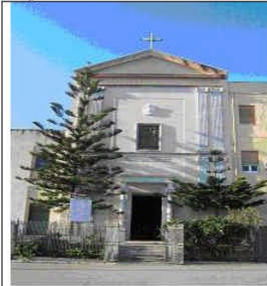
Figure 1 - Façade of the Shrine
